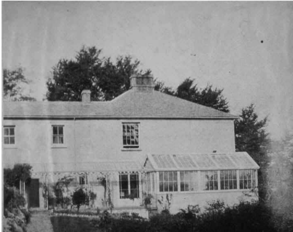
Last remaining section of Rosehill House
